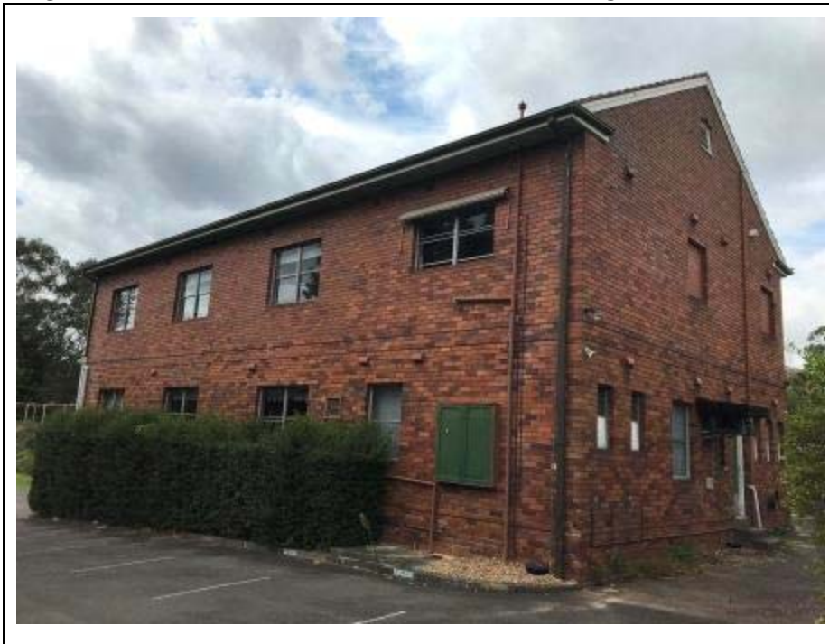
Image 6.2.1 View of northern side of clubhouse building
