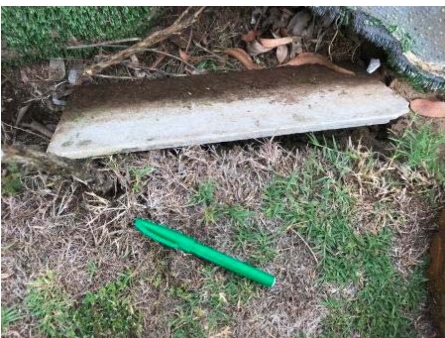
Image 6.10.4 View of fibrous cement sheeting along edge of bowling green
